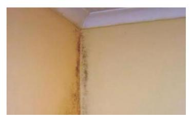
Mould behind a wardrobe. Condensation has settled on a cold outside wall, the lack of air movement because the free standing wardrobe allows mould to grow unchecked. Black marks above skirting boards and behind beds is another area black mould gathers, a bed situated close to the wall hinders air flow.
