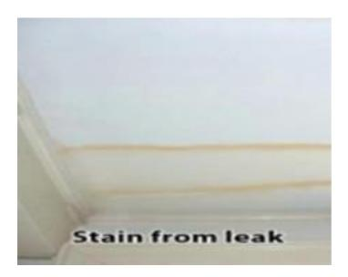
A Water stain on the ceiling. A large but typical water stain on a ceiling, the brown tea colouration is the hallmark of a leak as compared to the black mould or shadowy look of a condensation mark. This holds true in 80% of cases. Below shadowy wet look of condensation and mould.
